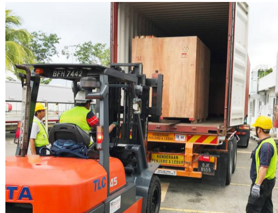
NVOCC (Installation of facility equipment )
