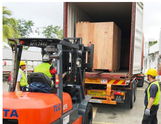
NVOCC (Installation of facility equipment )
