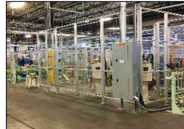
On site machine Installation
